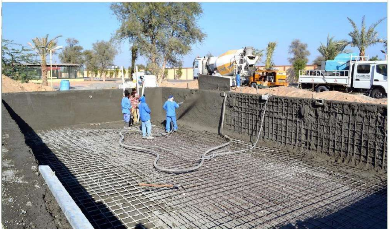
CONSTRUCTION OF A POOL AT MADAM
